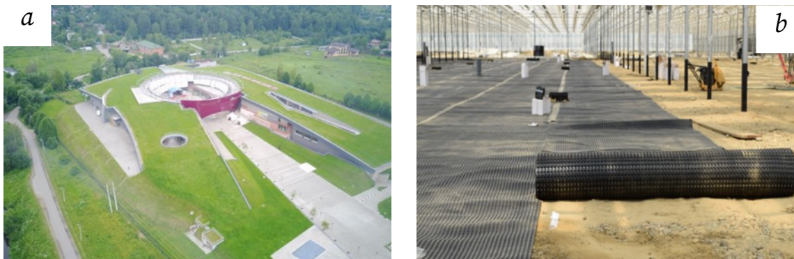
Fig. 6. Application of profiled membranes at real construction objects: a – the green roof of the museum complex; b – installation of floors on grade for a large agricultural complex
